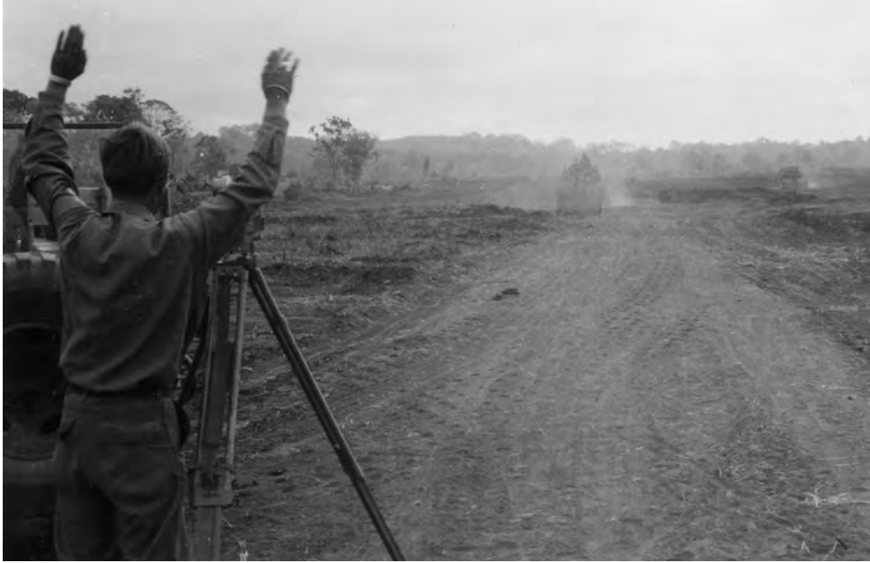
Surveying and site preparation at Duc Lap
